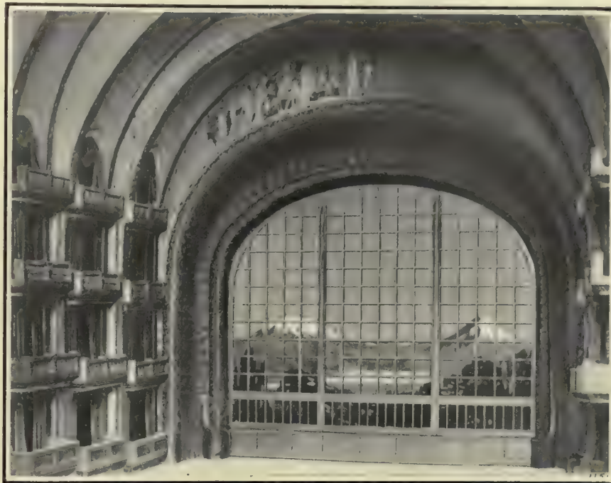
INTERIOR OF THE THEATRE SHOWING THE MOSAIC CURTAIN
